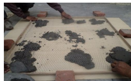
b. Laying of mortar
